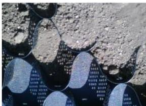
Sand infill in the GEOWEB cellular network remains confined and stable.
